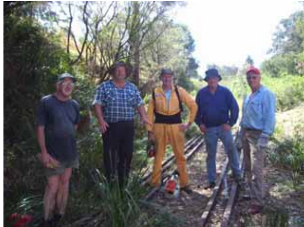
If there's a railway, there must be a work gang. This is the Dorrigo work gang.
