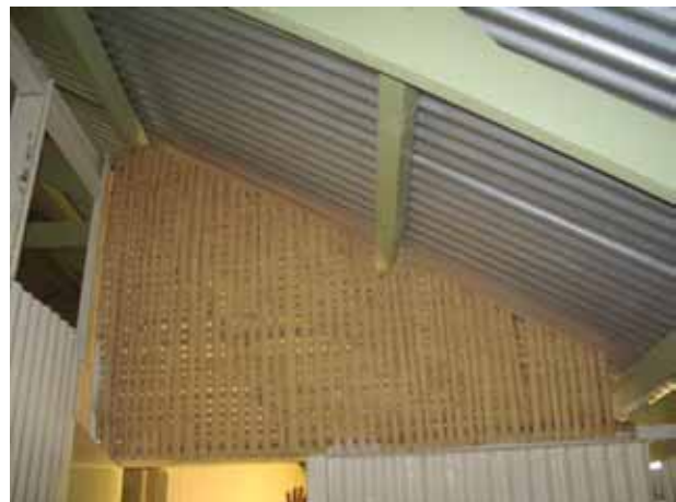
Bamboo screens were very popular in the early 1900s, and we have retained this sample which provides a screen yet allows air to circulate.
