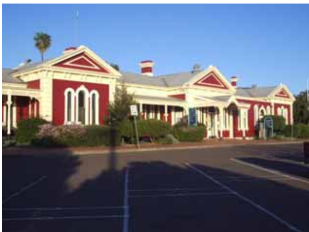
The magnificently restored Tamworth Railway Station.
