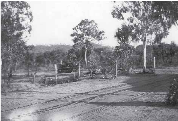
First Australian BIPOD Fuel Depot at present day Finlay Road, Adelaide River.
