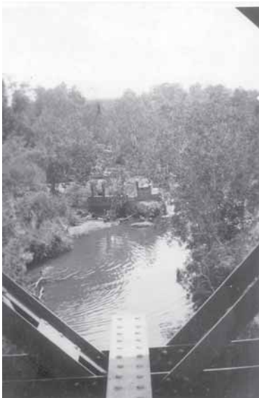
A great shot of the substantial remnants of the Verburg wier taken from the railway bridge in 1942. Note the low level bridge being built in the background. It's rumoured that the Army destroyed the wier and this photo suggests that the Army may well have 'cleared it up a bit' to protect the new bridge. It appears that the railway bridge had not been decked for Wet Season use by road traffic.
