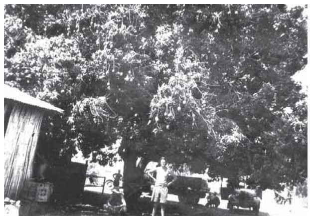
The original cook house and mess. Check out the size of the mangos on that tree!
